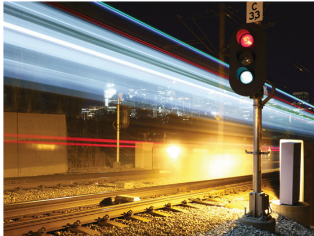
FIGURE 1: Today's railway racks need to optimize space as much as the electronic components themselves.
